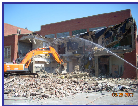
Figure 0.3 - Demolition of Terrell Junior High
