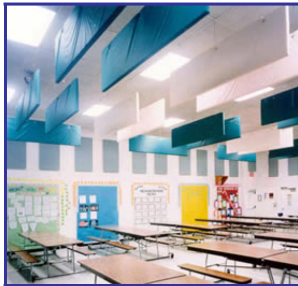
Figure 3.9 - School with Acoustical Wall Panels
